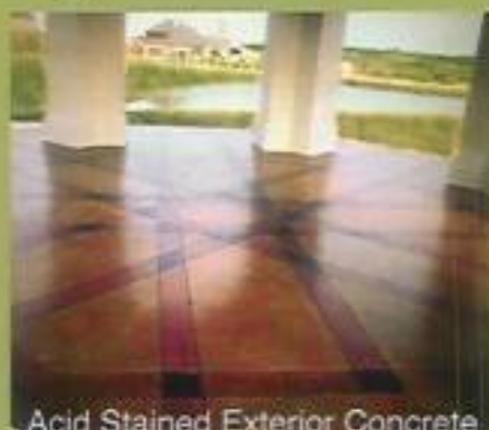
Acid Stained Exterior Concrete
